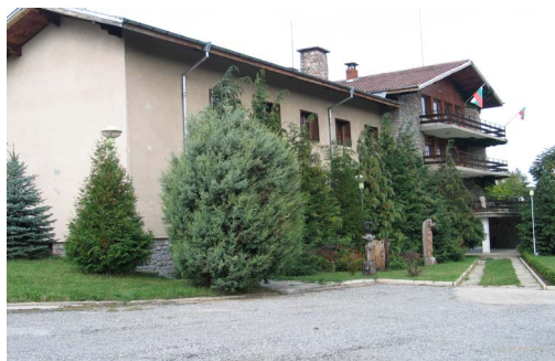
The building of the Petrohan training and experimental forest range, Barziya village.
