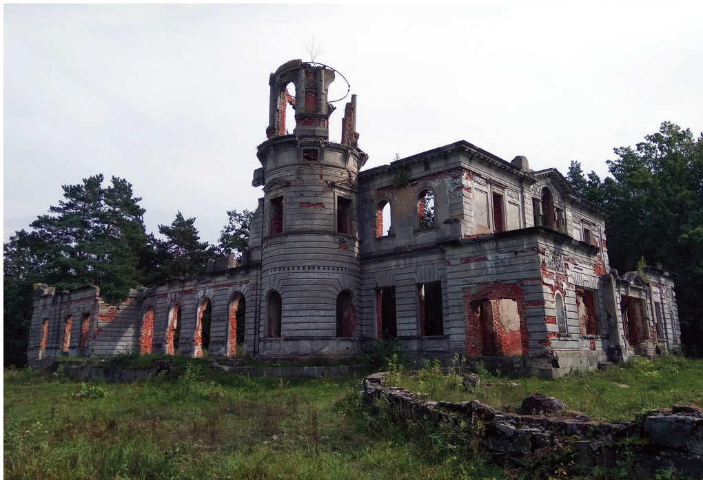
Fig. 2. The current state of the estate in the village Denyshi. (co-ordinates 50°12'19.03"N, 28°24'44.29"E)
